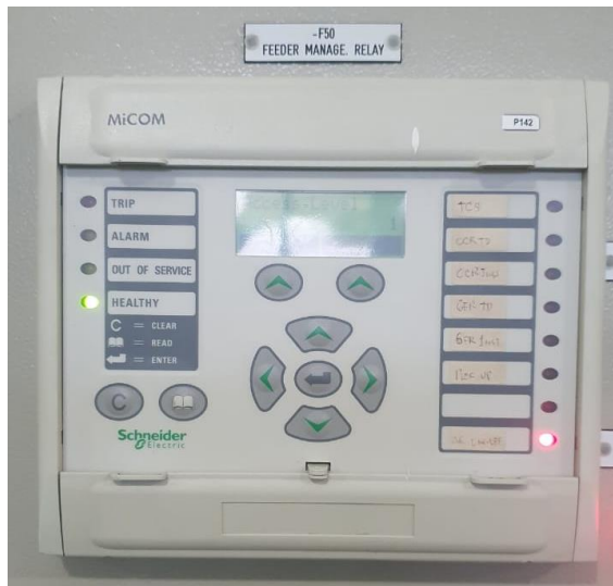
Gambar 4.4 Relay Proteksi OCR/GFR Micom P142
