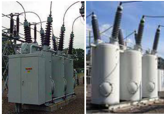
Gambar 2.5. Oil Circuit Breaker
