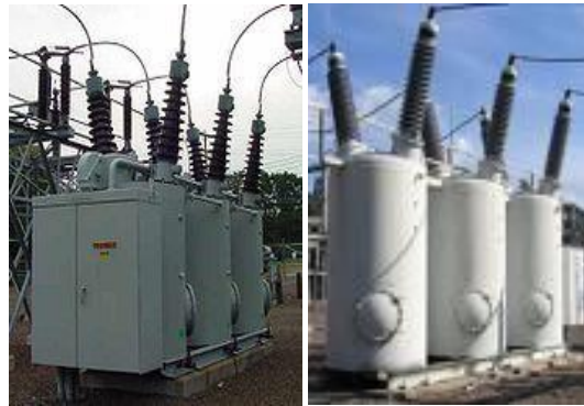
Gambar 2.5. Oil Circuit Breaker
