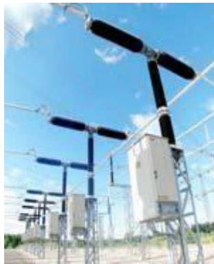
Gambar 2.10. SF 6 Gas Circuit Breaker
