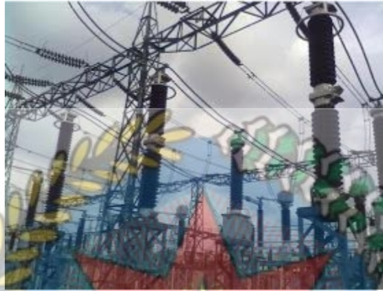
Gambar 2.8. Lighting Arrester GI
