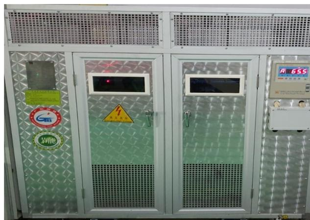
**Gambar 2.34 Exciter Transformer PLTA Wampu**
