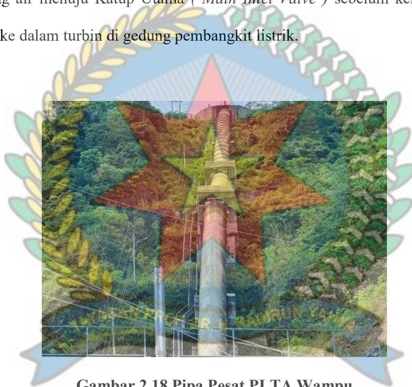
**Gambar 2.18** Pipa Pesat PLTA Wampu
